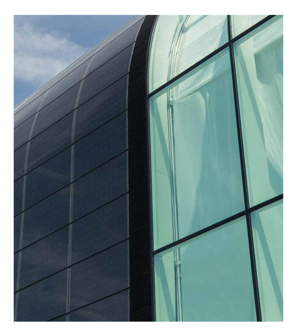
A mix of triple glazing and a unitised curtain wall with outstanding thermal characteristics significantly reduces heat loss via the façade and results in a U-value below 1.0 W/m<sup>2</sup>k.
