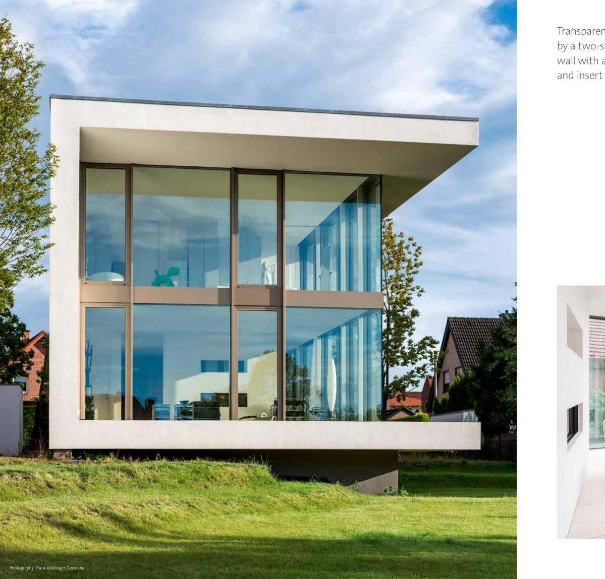
Transparency was ensured by a two-storey high curtain wall with anodised profiles and insert elements.
